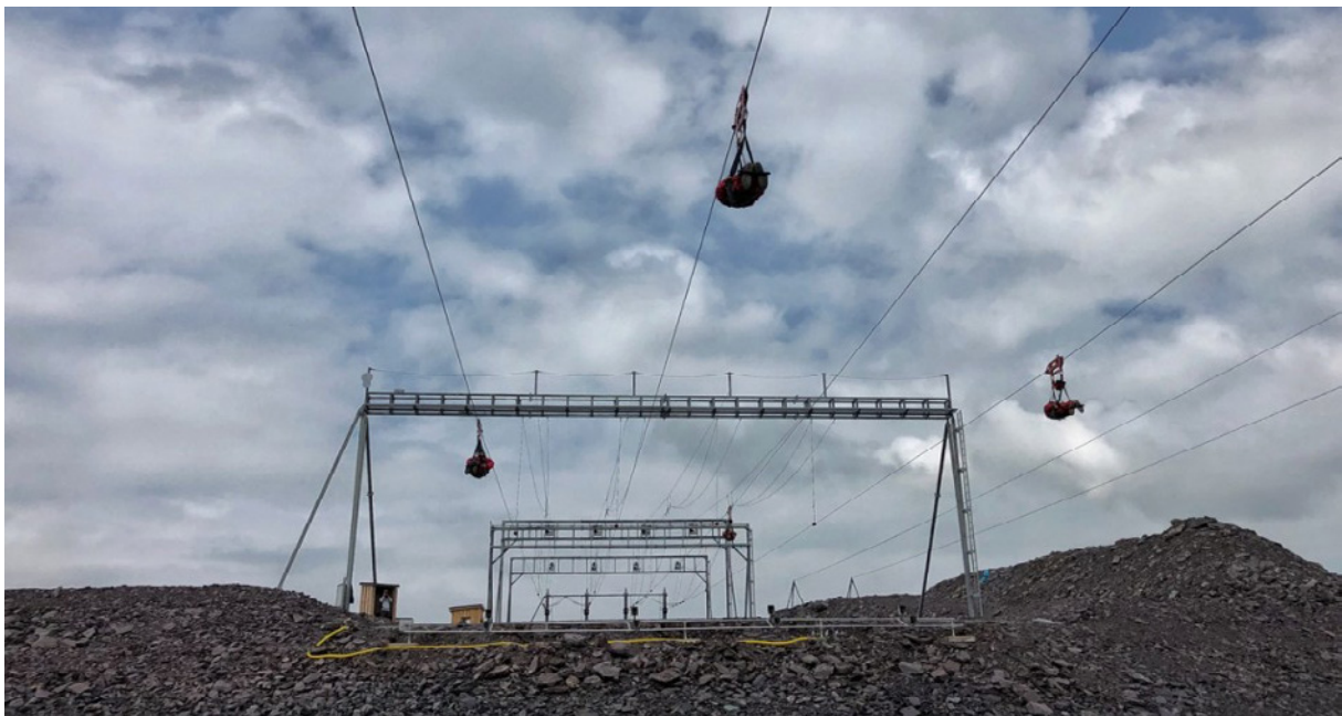
Indicative galvanised steel gantry like that found at existing Zip World locations
