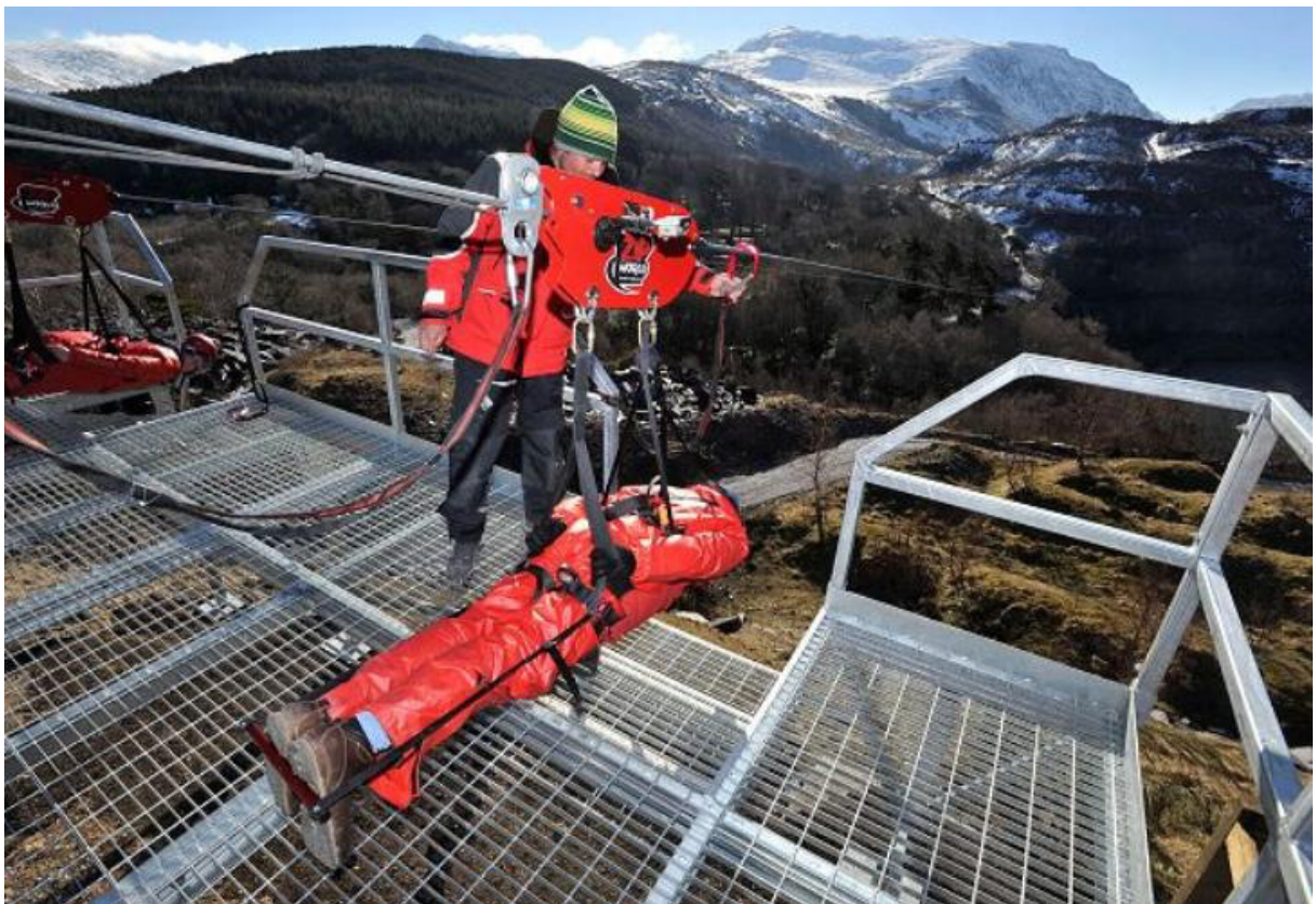
Galvanised steel grate flooring and stairs with key clamp and mesh guardings
