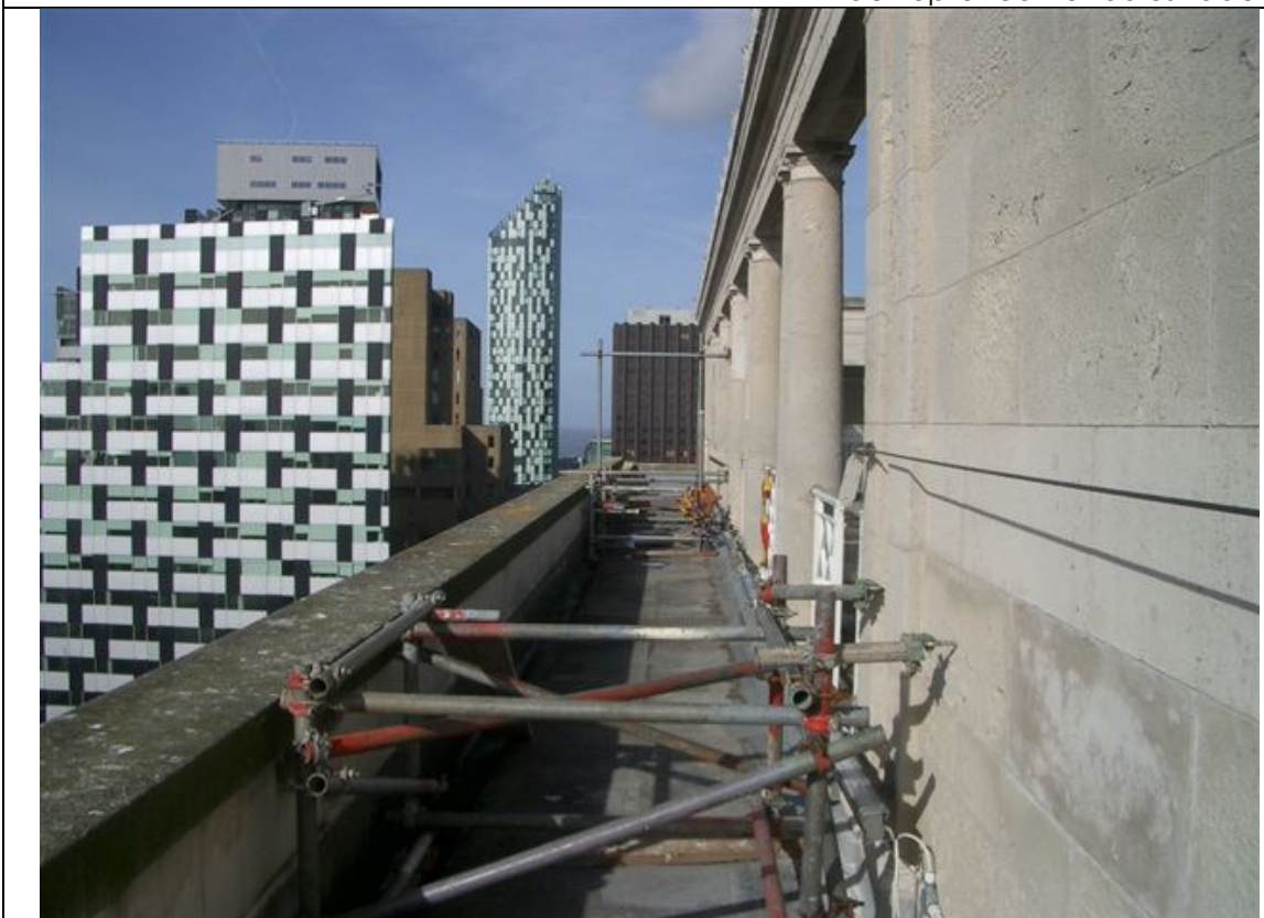
Supports to mock up of end panel and centre T panel balustrades
