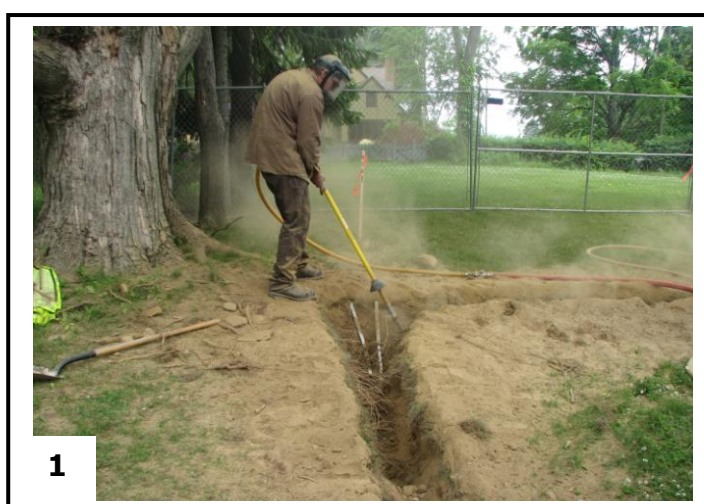
Picture 1: This shows the excavation process using an Air Spade
