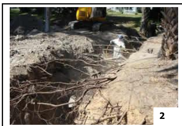
Picture 2: This shows the process of hand excavation below the root zone following the exposure of roots using an Air Spade
