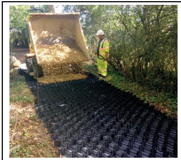
Installation of ProtectaWeb™ on site
