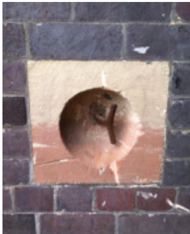
Cleat in reveal of loading bays
