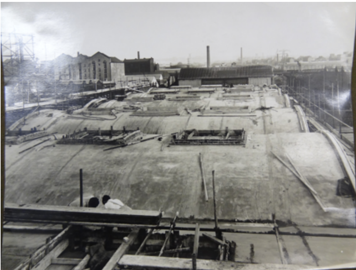
Work on barrel vaulted roof of Rum Warehouse around 1953 (c) MDHC
