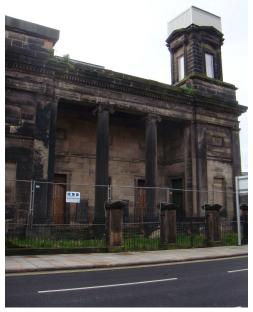
the retention of the remaining external walls of the principal church building and the construction of an internal steel frame in which will be constructed five floors of student accommodation around an open central courtyard.
