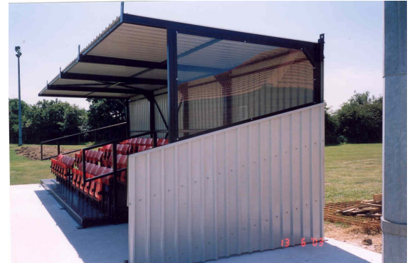
Full End Enclosure with Lexan Polycarbonate Glass at Viewing Level
