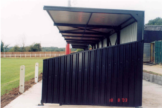
Side Enclosure Up to Handrail Level
