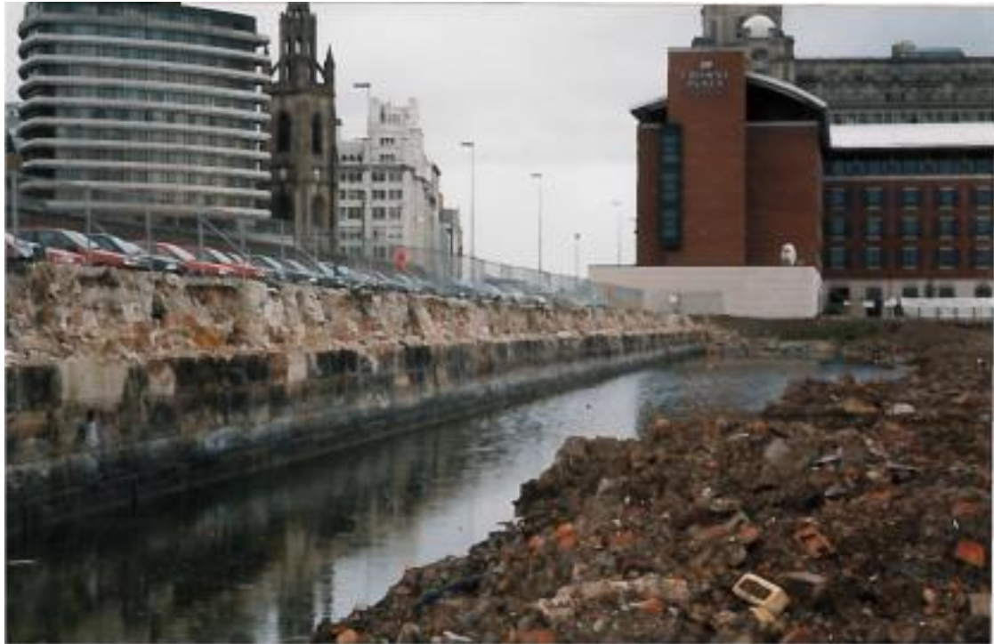
Photo 2.3: 1999 – dock wall exposed following break down of staging and begin of dock infill
