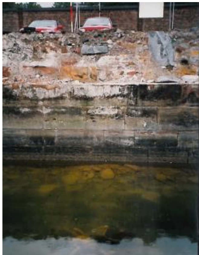
Photo 2.2: 1999 – dock wall exposed following the break down of staging
