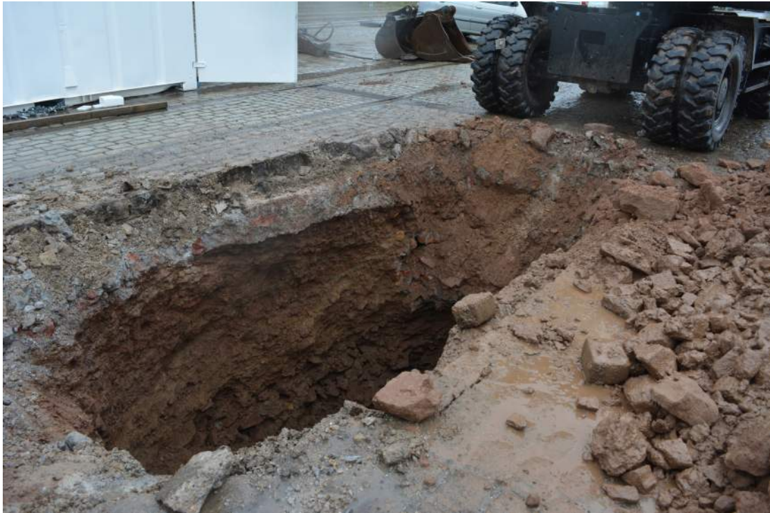
Plate 10. TT306. Brick lined culvert exposed in southern edge of trench. View looking south-east.
