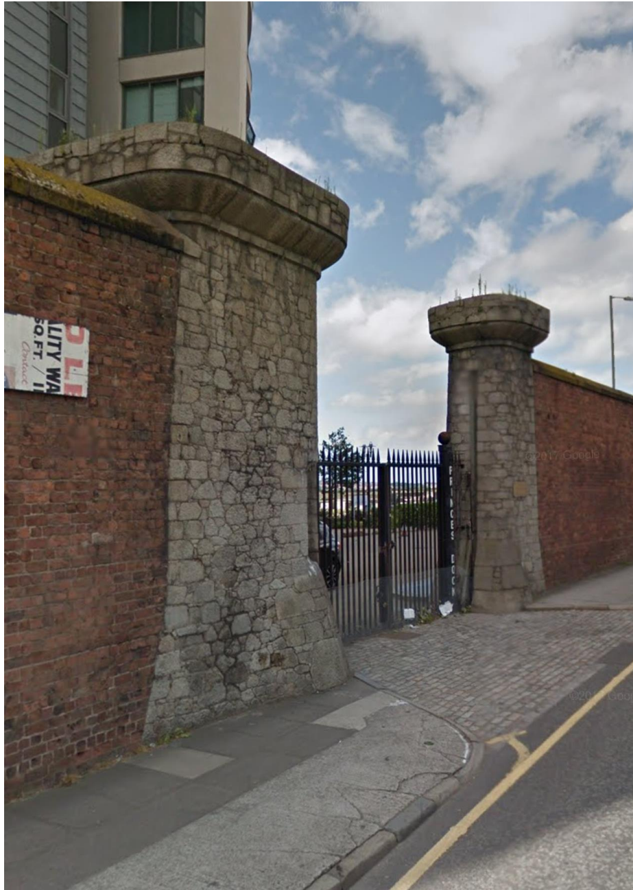
Figure 13- northern gateway to Princes Dock. These appear to be based on Hartley's dock gate designs from the 1840's, but date from the 1860's.
