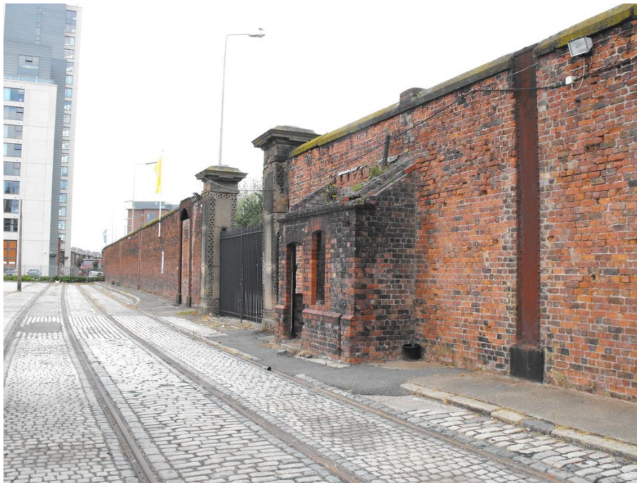
Figure 16- West of Dock Wall- note iron stanchions for supporting the later Liverpool Overhead Railway, and the former police hut (now re-roofed and stabilized).
