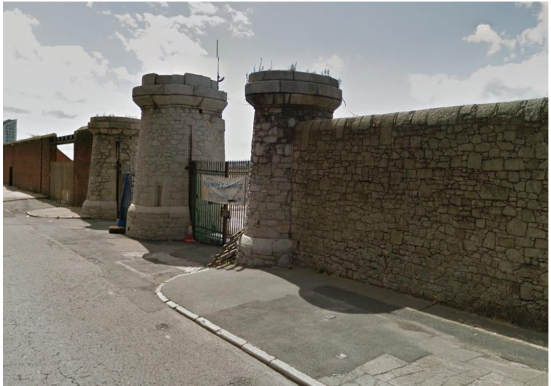
Figure 10- Entrance to Collingwood Dock, showing transition to granite for the gateways and walls.
