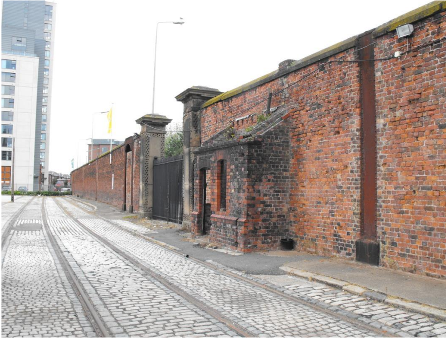
Figure 16- West of Dock Wall- note iron stanchions for supporting the later Liverpool Overhead Railway.
