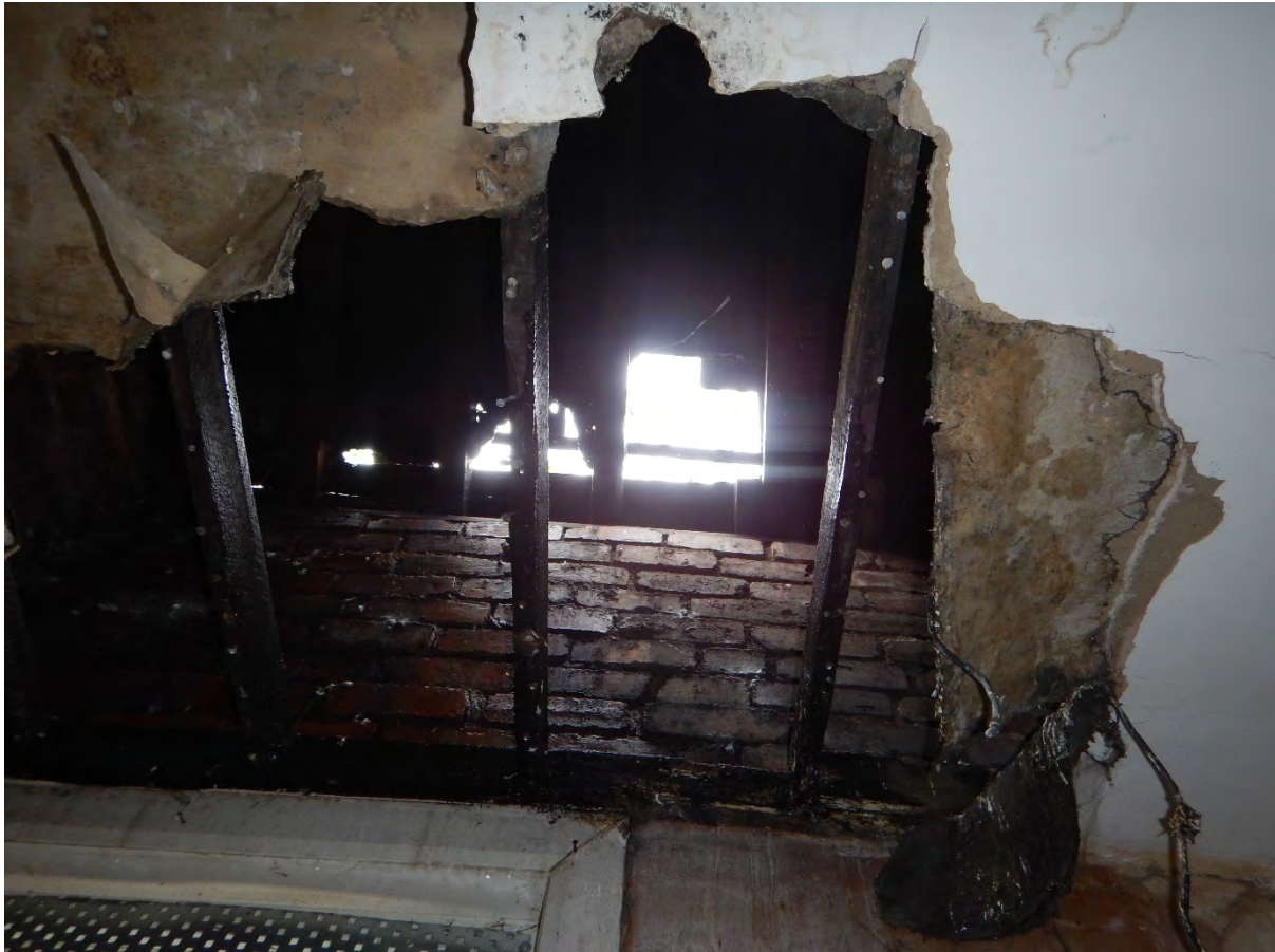
3.1a – A typical section of ceiling and roof void, now open to the elements, where ceilings have collapsed.
