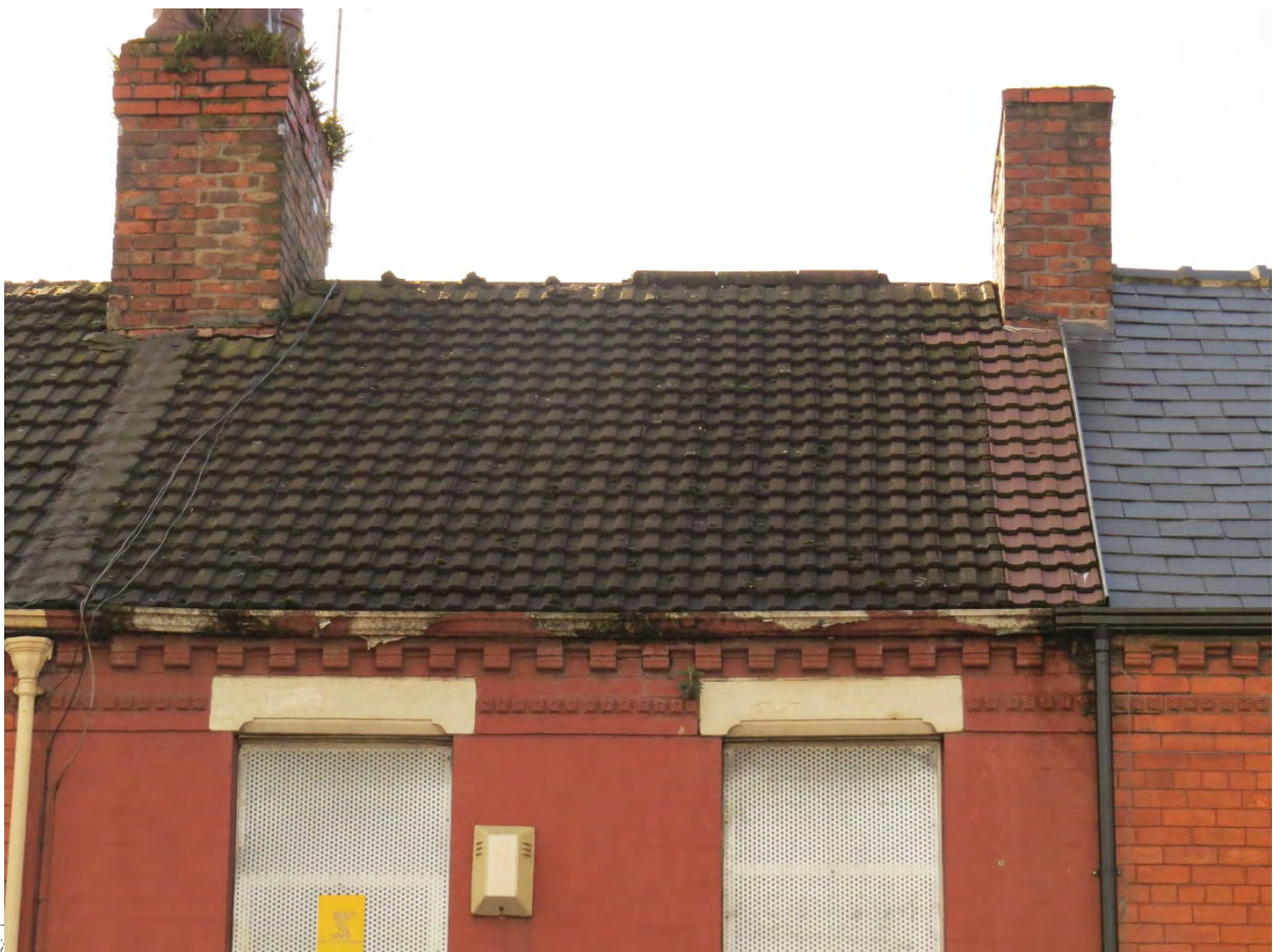
4 – Roofs are a mixture of slate and Marley tiles, many ridge tiles are missing.
