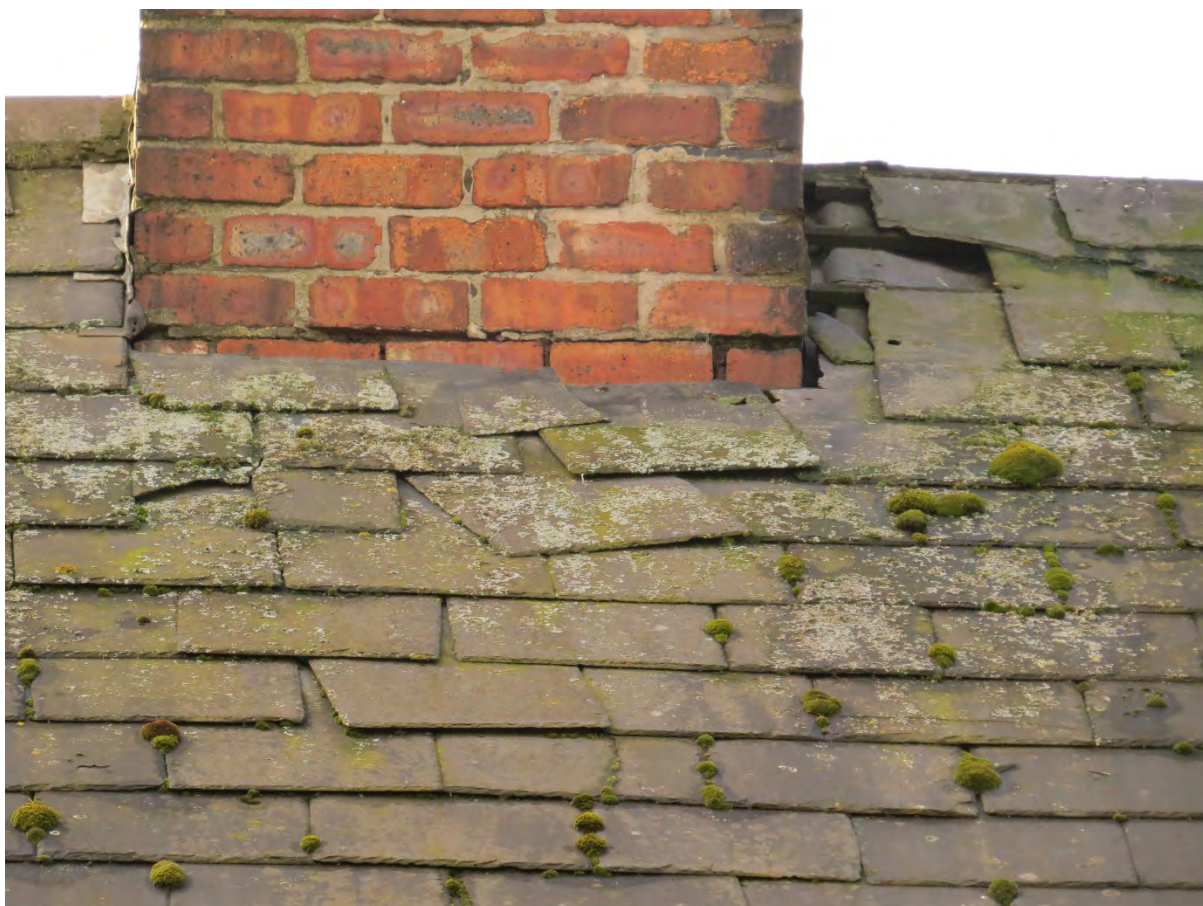
5 – Roof and ridge tiles have been disturbed where leadwork has been removed.
