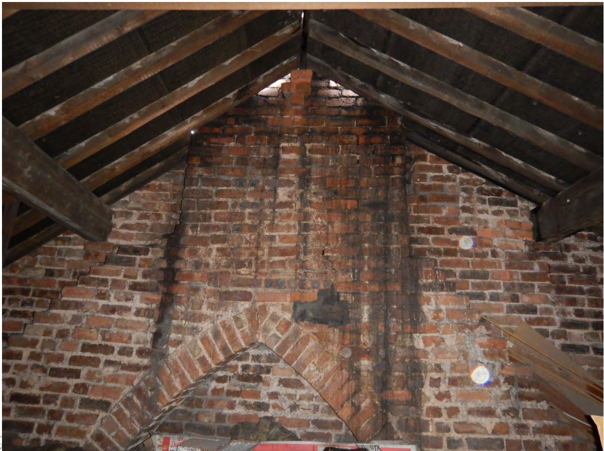
8 – Water is running down walls where leadwork and ridge tiles have been removed.
