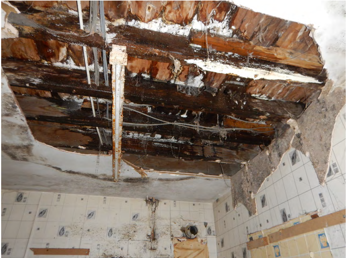
9 – The walls and floors are rotten as a result of water ingress.
