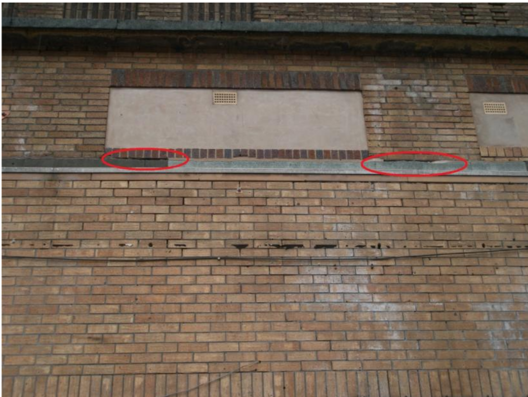
Figure 3h: Feature 5b – gaps in pointing on west face of structure.
