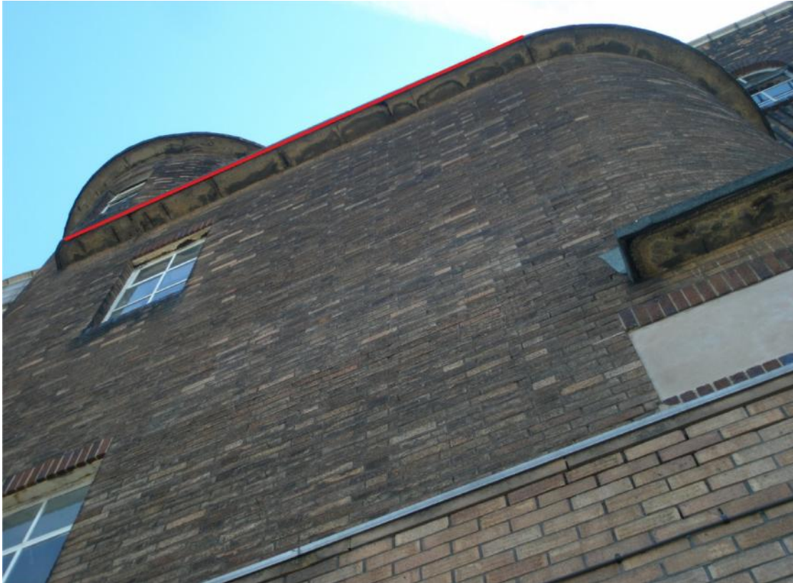
Figure 3c: Feature 2a – stonework overhangs on the north and west face of the structure show signs of weathering with potential gaps – see also Figure 3e.
