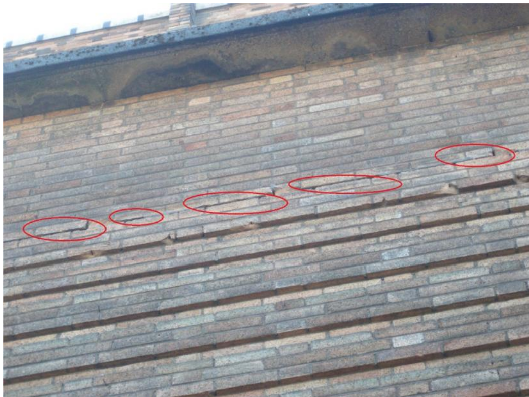
Figure 3b: Feature 2 – located on the north aspect of the structure, gaps in brickwork where pointing has eroded.
