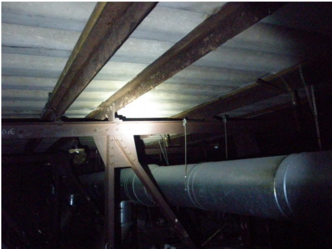
Figure 6j: Image 10 – this image shows the roofing material to the structure which appears to be corrugated asbestos and not metal as suggested in the Preliminary Ecological Appraisal.
