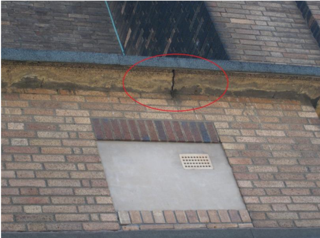
Figure 3e: Feature 4 – close up of crack in stonework overhang on the west face of the structure. There are similar overhangs on the north face of the structure which may also have potential roosting opportunities for bats.
