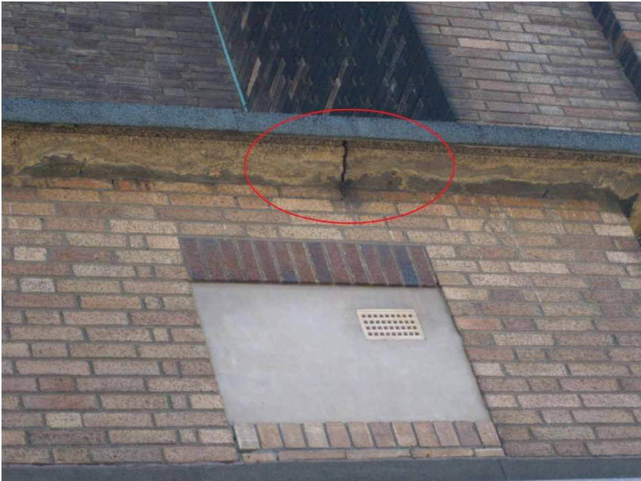
Figure 7: showing crack in cement rendering on the west aspect of the structure providing potential roosting opportunities for crevice dwelling bat species.
