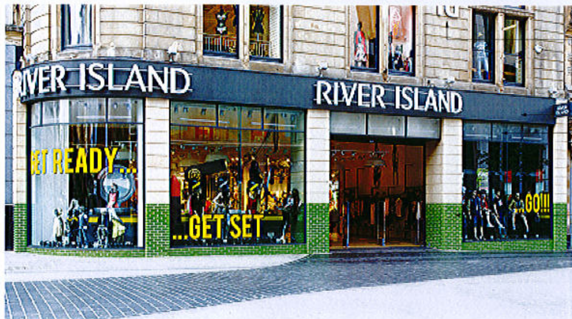
EXISTING SHOPFRONT PHOTOGRAPH
