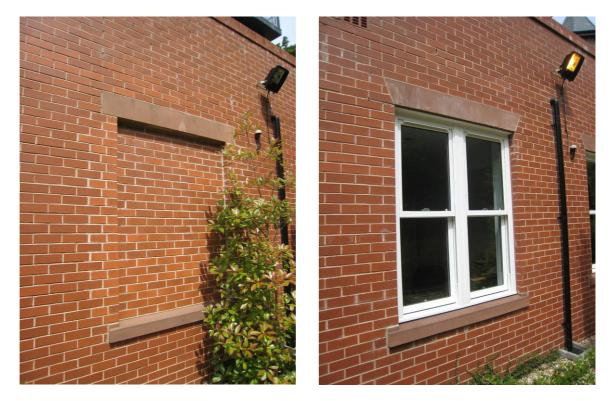
The large access door into the existing The Glen storage area will be infilled with facing brickwork which will contain a new window as illustrated on the proposed elevations.
