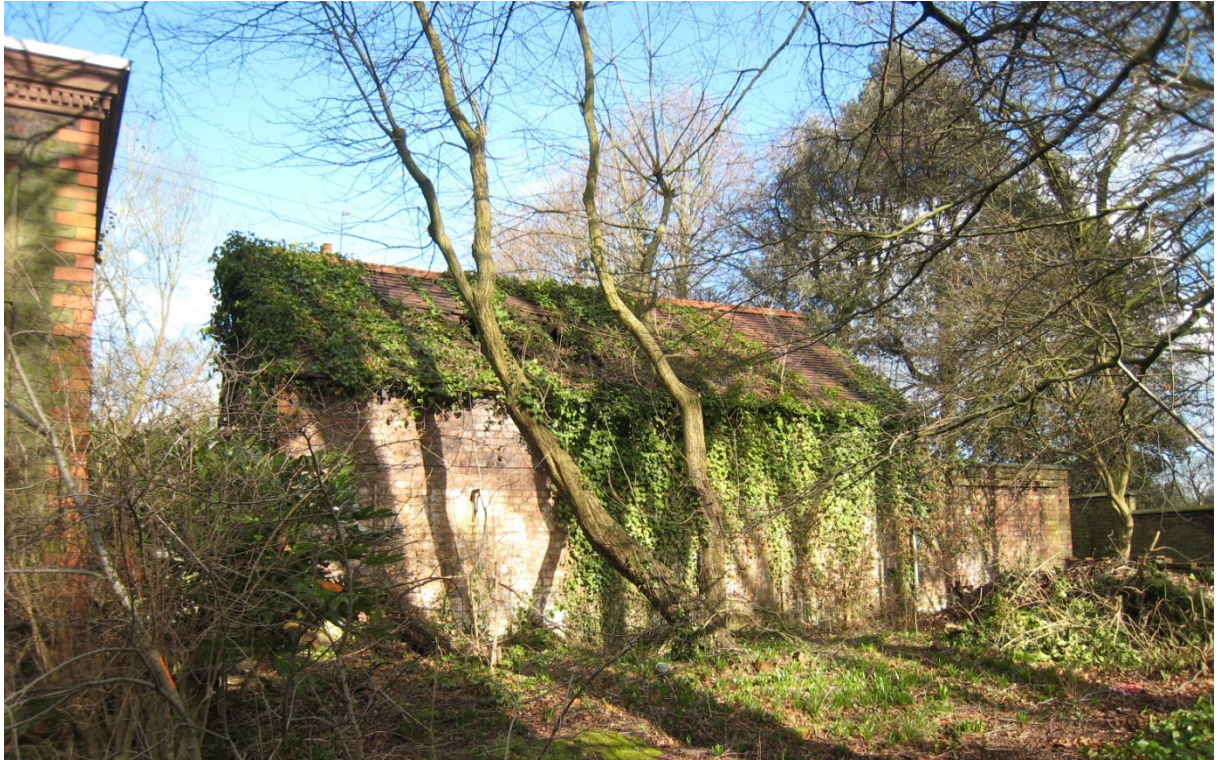
Garage building with hole in roof and threatened by unstable tree.
