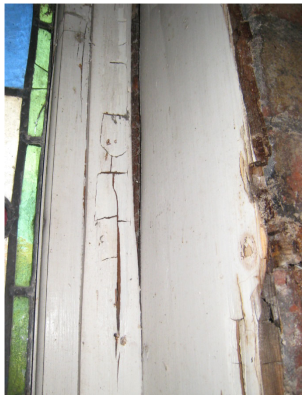
Cuboidal cracking in window frame.
