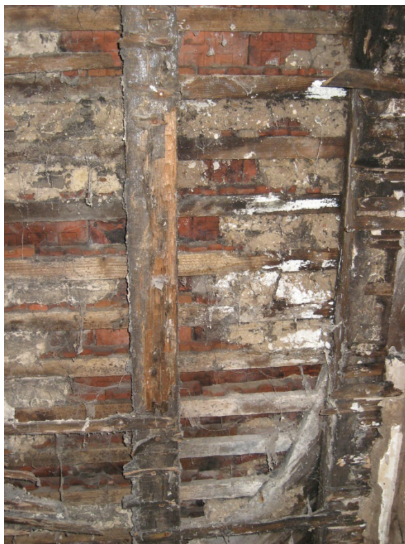
Rafters, roof battens and tiles.
