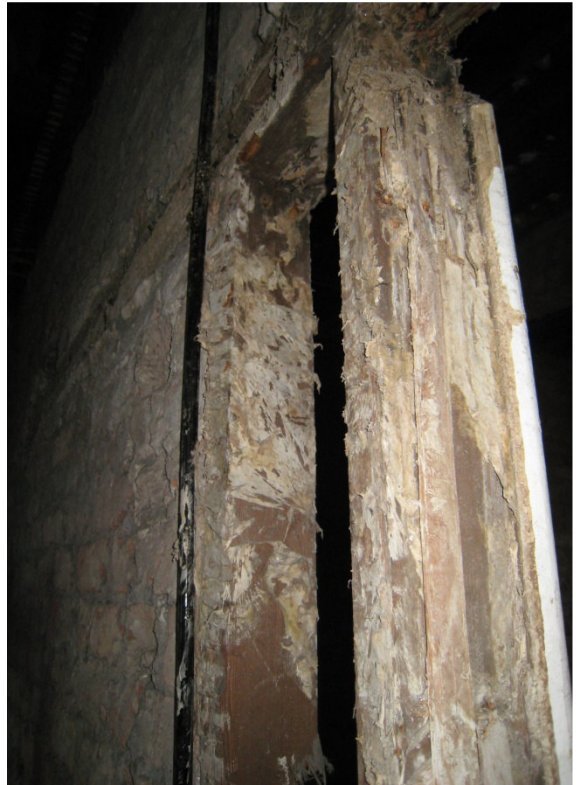
Mycelium from dry rot in stud wall.
