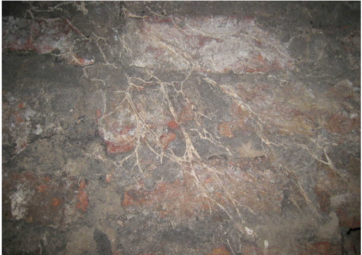
Dry rot strands which would have been behind plasterwork.
