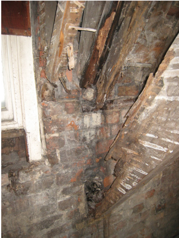
Truss foot destroyed by dry rot.
