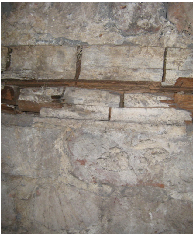
Cuboidal cracking in dry rot affected timber.
