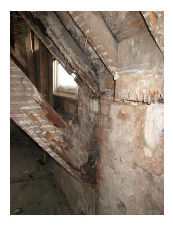
The ground and second floor properties have been uninhabitable for a substantial number of years and unfortunately, a lack of any meaningful maintenance has meant that the building has not remained weathertight and this has resulted in water ingress in numerous areas for what appears to have been extensive periods. It is clear that repairs have not been promptly carried out or in some cases not at all and if so not to a satisfactory standard.
