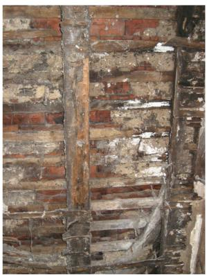
Ingress of moisture has evidently provided ideal conditions for dry rot to become established. Signs of dry rot are apparent to a number of timber and masonry areas. Also, above the main staircase there has been a leak from the roof and both landings are decaying along with the roof timbers.
