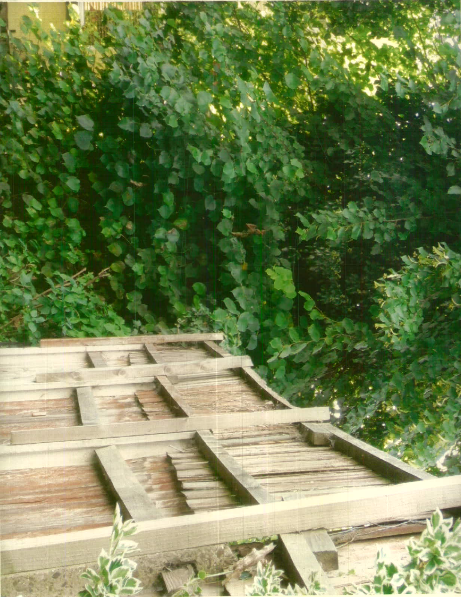
tree closely hugs fence and hangs over alley way to cragside back garden! Photo 2
