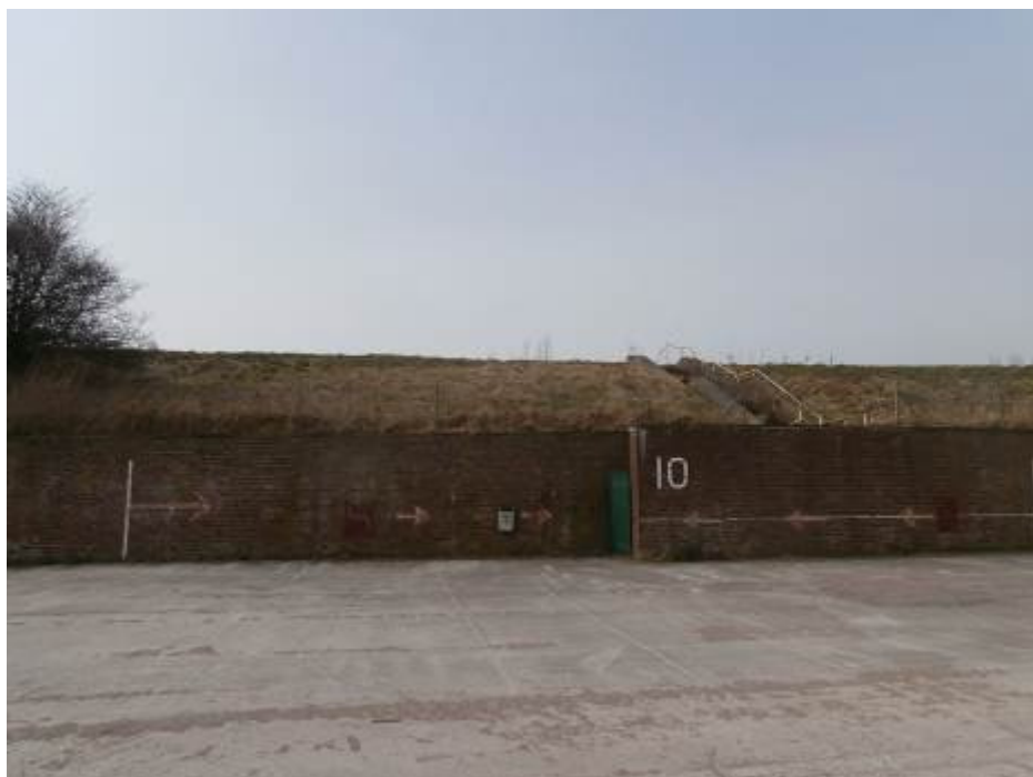
PLATE 12: THE EXISTING RETAINING WALL ON THE TENNIS COURTS RETAINING THE LANDFILL MATERIAL.
