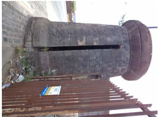
LEFT: Last remaining existing Timber Sliding Gate at Stanley Dock. Full Restoration to be carried out and reinstated. RIGHT: Granite Pier Sliding Gate Access through. To ensure completely clear of debris and any brick infill.
