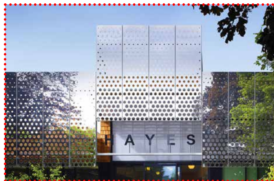
Perforations in metal cladding
