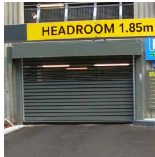
6. Vehicle roller shutters
