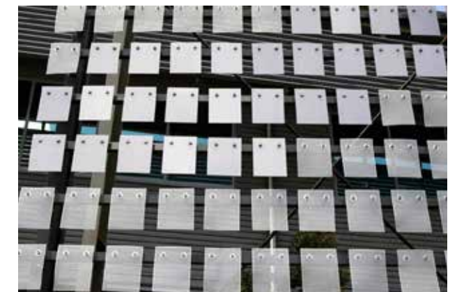
4. Naturally ventilated facade in lightweight opaque material
