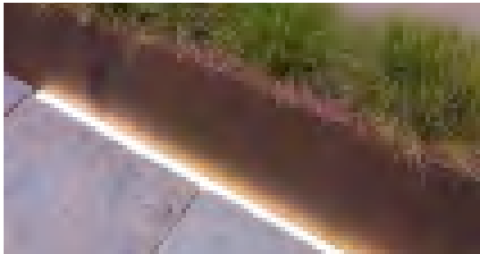
Feature strip uplighting to planter edges
