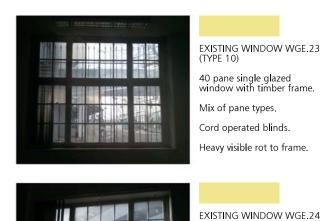
40 pane single glazed window with timber frame. Heavy visible rot to frame.
