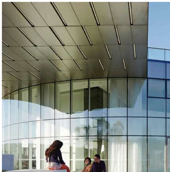
02 Horizontal rainscreen soffit.
