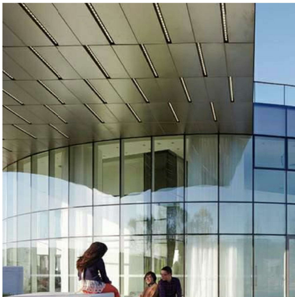
02 - Horizontal rainscreen soffit.
