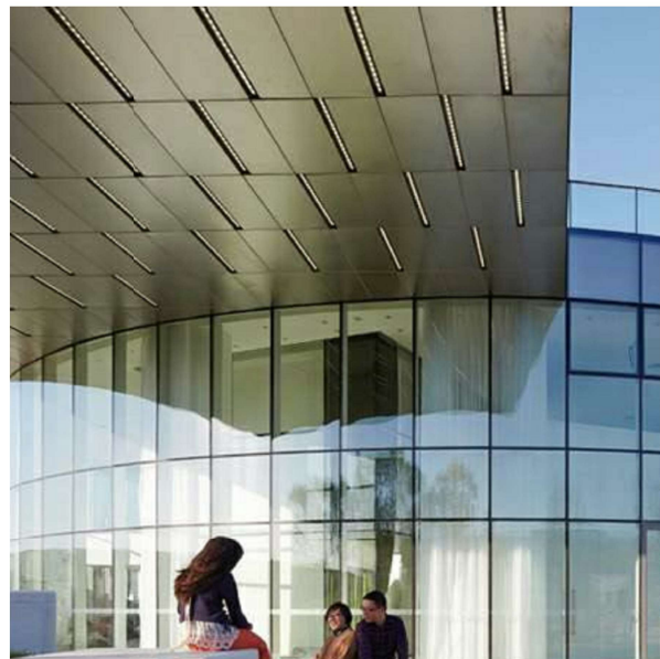
02 - Horizontal rainscreen soffit.
