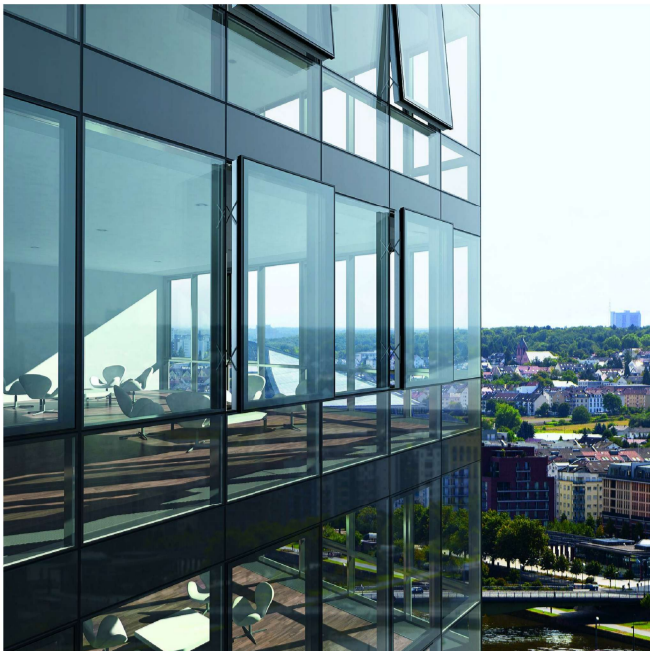
01 Capless / Unitized Glazing System with fritted glass. System to intergal fins / solid, openable panels
