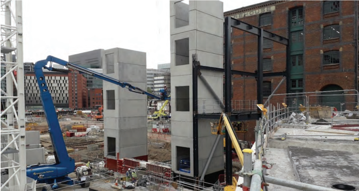
Typical precast concrete lift shafts, overview and built examples
