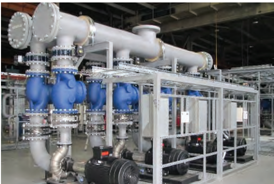
Example modularised MEP plant skids
