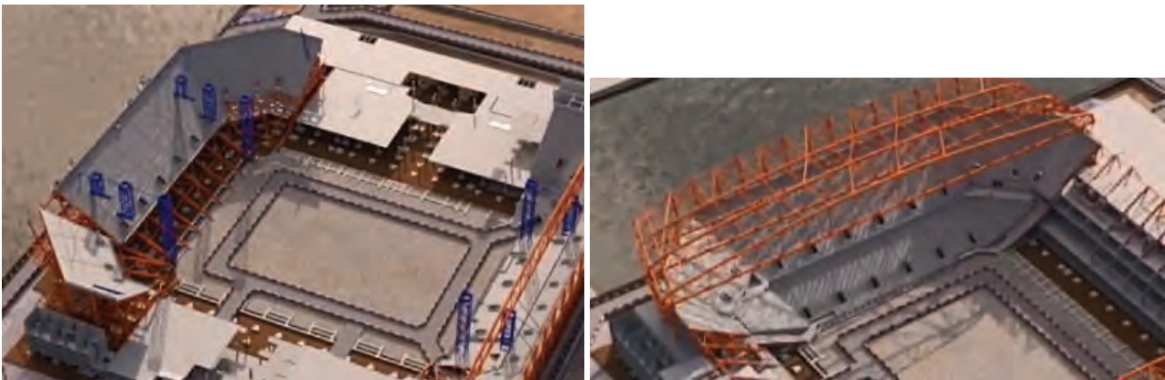
Images showing phased install of terracing on south stand pre & post trestle removal
