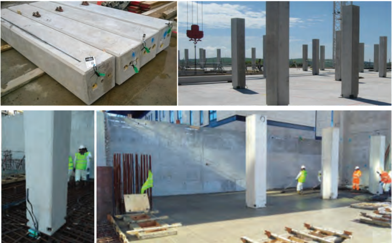
Precast columns before and during installation at West Cumberland Hospital
