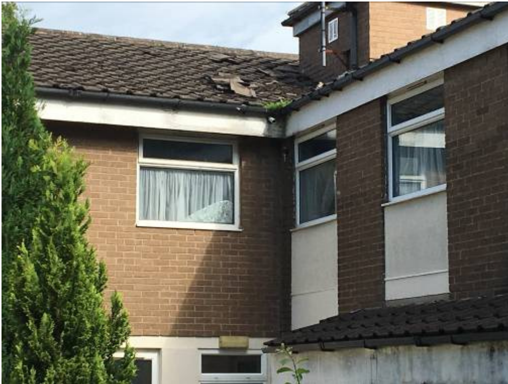
B1 Missing & loose roof tiles (East elevation)
