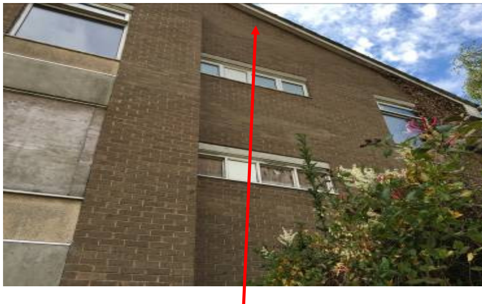
B2 gaps at soffit boards (north elevation)
