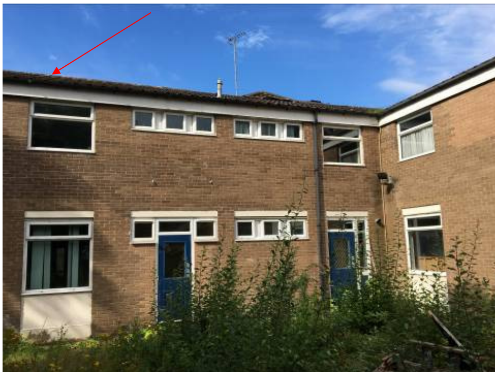
B1 gaps at roof tiles (East elevation)
