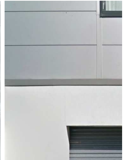
Metal Cladding and Render
