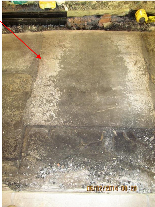
Figure 2 - Yorkstone Slabs exposed as part of previous works on existing platform 3
