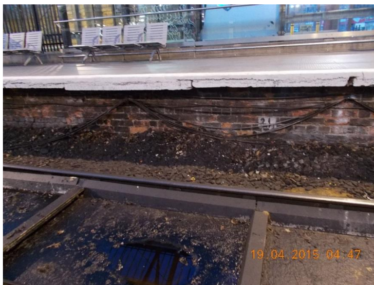
Figure 4- Existing platform 9 copers
