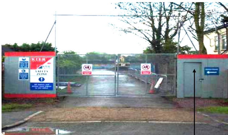
Kier NW Site Set Up: Secure Hoarding & Gated Entrance
