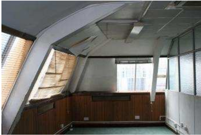
Mansard Roof at the 4th floor
