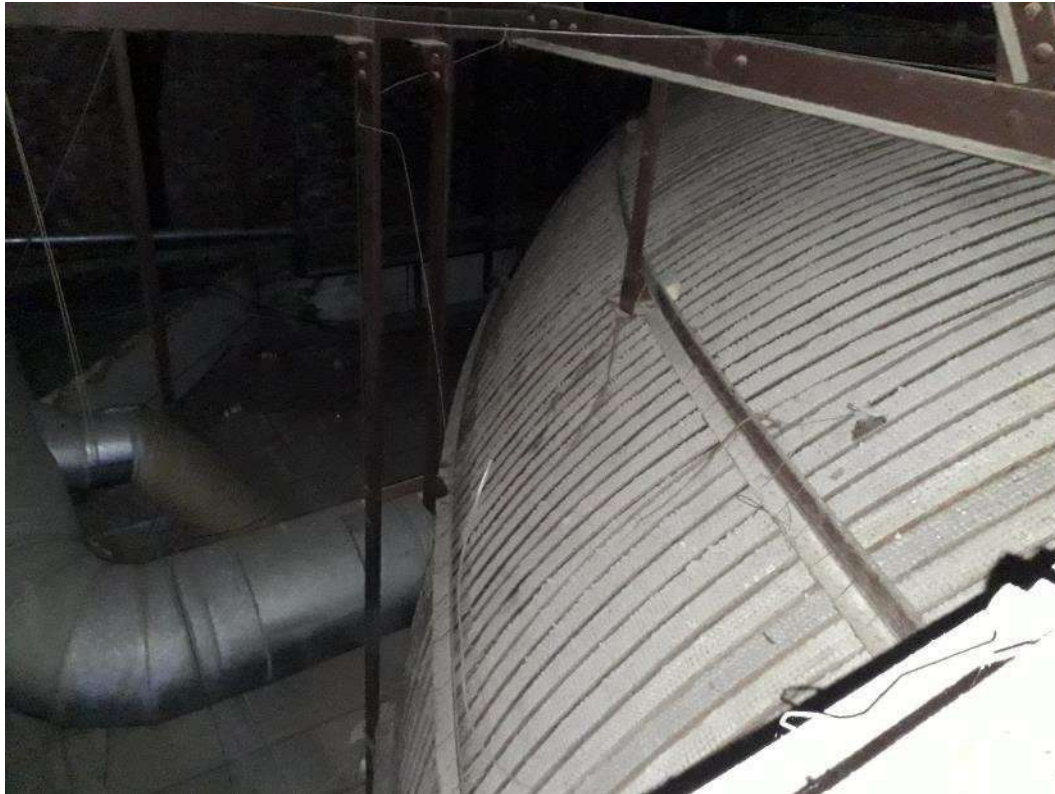
Plate 18 Image of extant original fibrous plaster ceiling on metal laths with the curved shape seen in plate 13 evident (Source: Space Architects June 2020)
