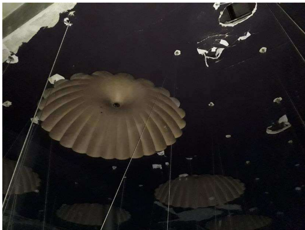
Plate 15 Image of extant scalloped plaster recesses in the ceiling above the modern suspended ceiling of the bingo/snooker hall (Source: Space Architects June 2020)
