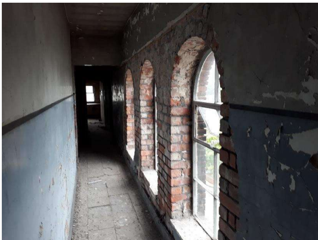
Plate 17 Image of existing western corridor at first floor with existing plasterwork and later metal windows (Source: Space Architects June 2020)
