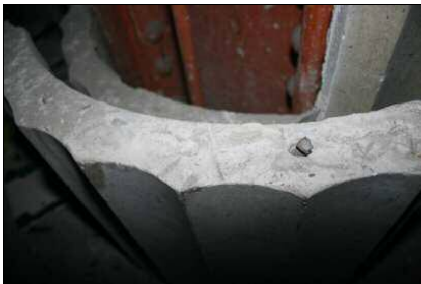
Casting with metal pin joint visible
