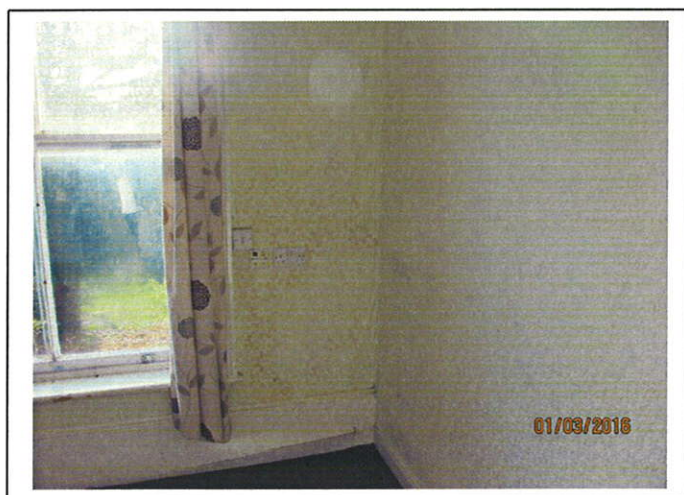
First Floor Room 6 - Damp penetration through the front wall.
