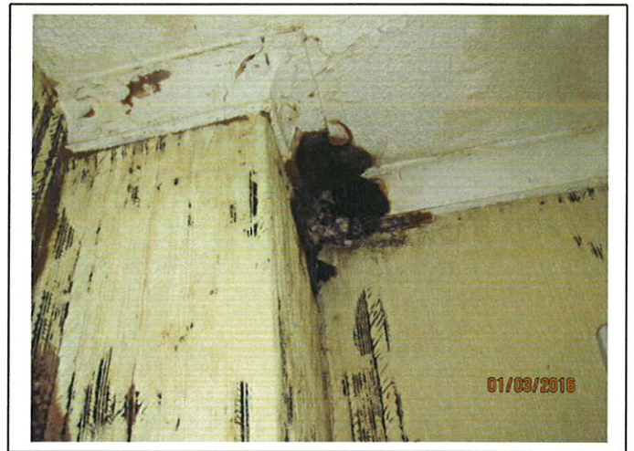
First Floor Room 14 - Damp penetration causing collapse to ceiling, mould growth in the en-suite.
