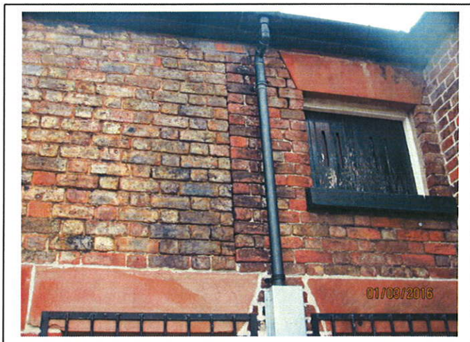
Joint in masonry.
