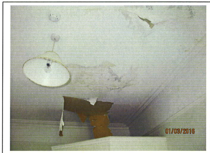
First Floor Room 1 - Damp penetration through the ceiling.
