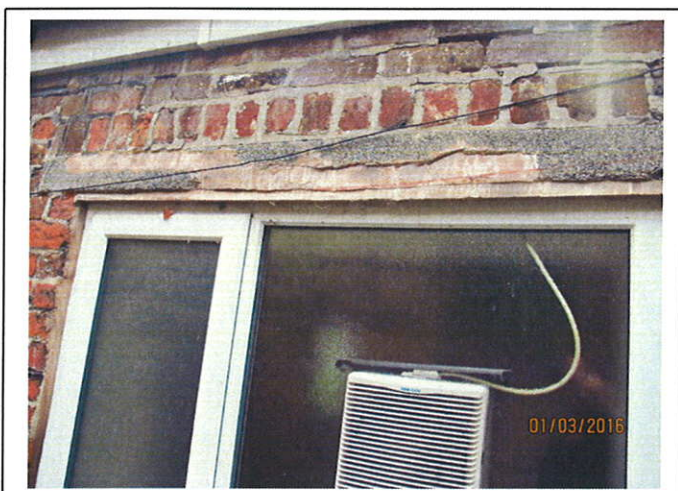
Spalling lintel on rear elevation.
