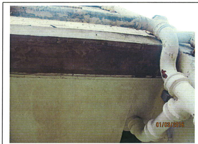
Spalled concrete lintel.
