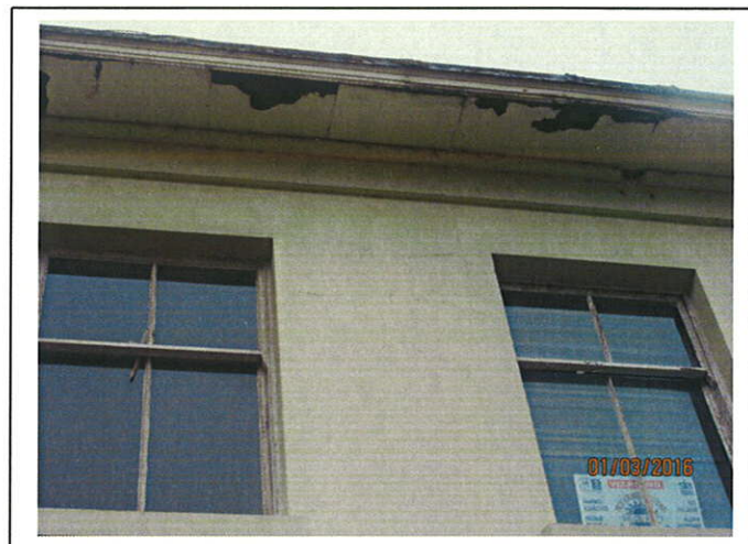
Rotten soffit boards.
