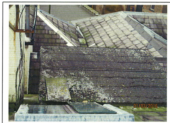
Main Roof - External Defects.
