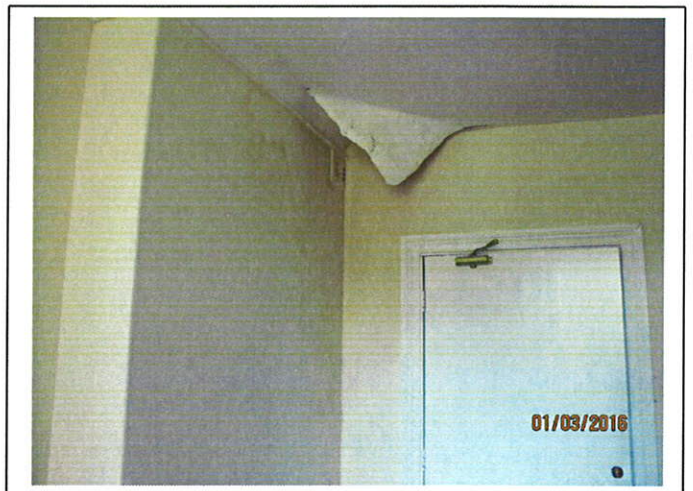
First Floor Room 15 - Leaking roof .
