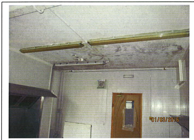
Ground Floor Room 19 - Damp in ceiling and fungal growth.
