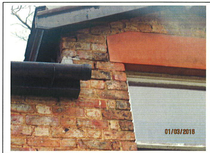
Slight movement at lintel end.
