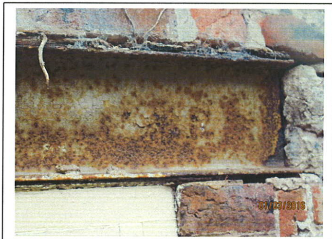
Corroded steel over window in rear elevation.
