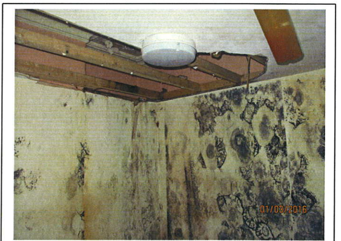
First Floor Room 20 - Collapsed ceiling and mould growth
