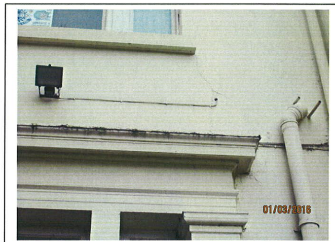
Typical cracking in render.
