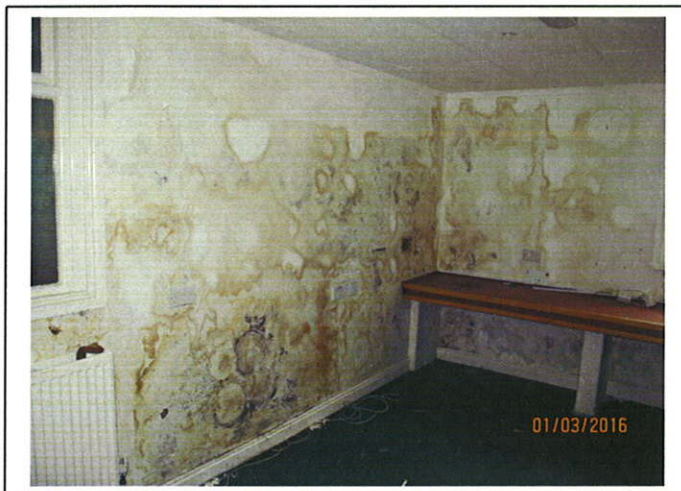
Basement Room 2 - Damp penetration through retaining walls
