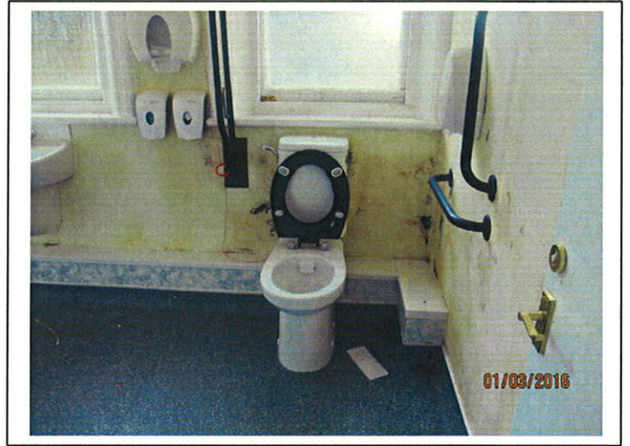
Ground Floor Room 15 - Damp penetration through side wall
