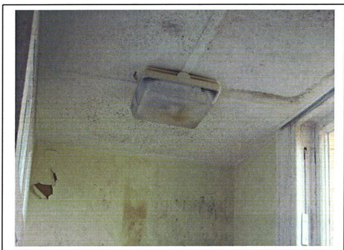
First Floor Room 10 - Damp penetration and mould growth.
