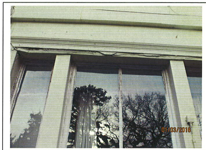
Front Elevation - Cracking over feature window.
