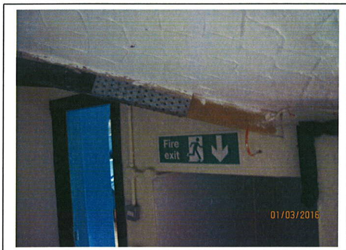
Splice repair to valley beam.
