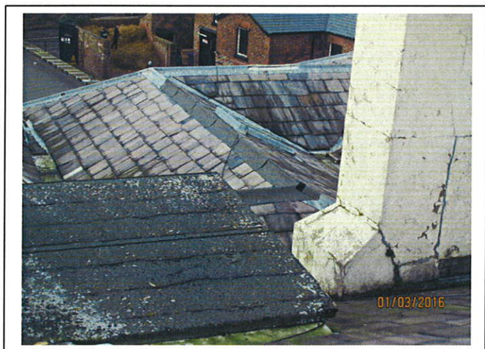
Main Roof - External Defects.
