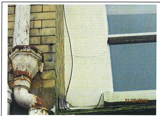
Left hand elevation - Cracking in render.
