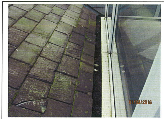
Main Roof - External Defects.
