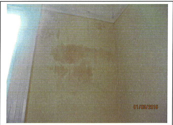
Ground Floor Room 9 - Typical damp penetration through from wall.
