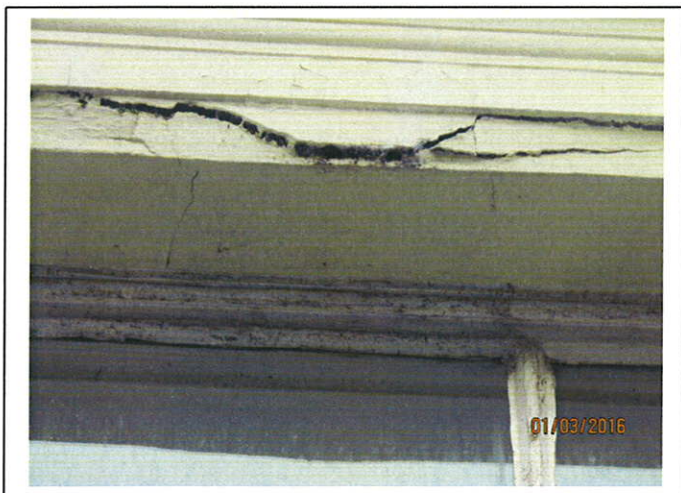
Front Elevation - Cracking over feature window.
