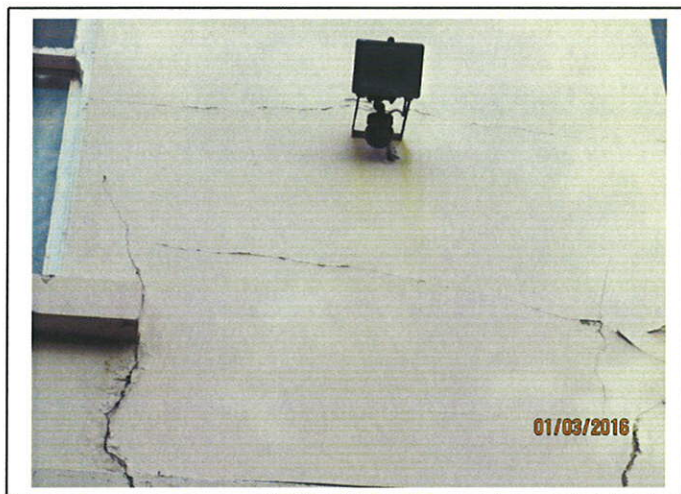
Front Elevation - Typical cracking in render.
