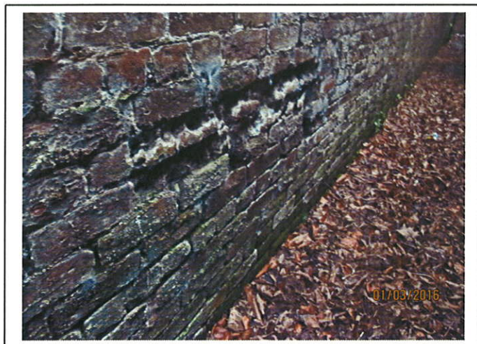
Rear Elevation - Spalled masonry.
