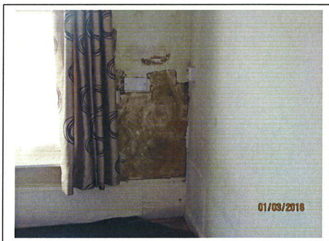
First Floor Room 7 - Damp penetration through the front wall.
