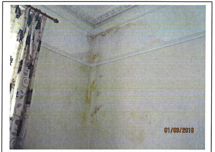
Ground Floor Room 10 - Damp penetration through front wall and side wall
