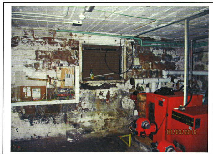
Basement Room 10 - Damp penetration through retaining wall
