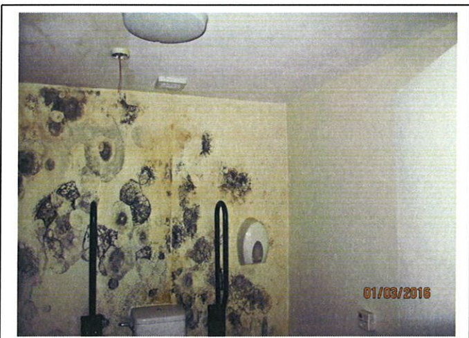
First Floor Room 20 - Mould growth on walls
