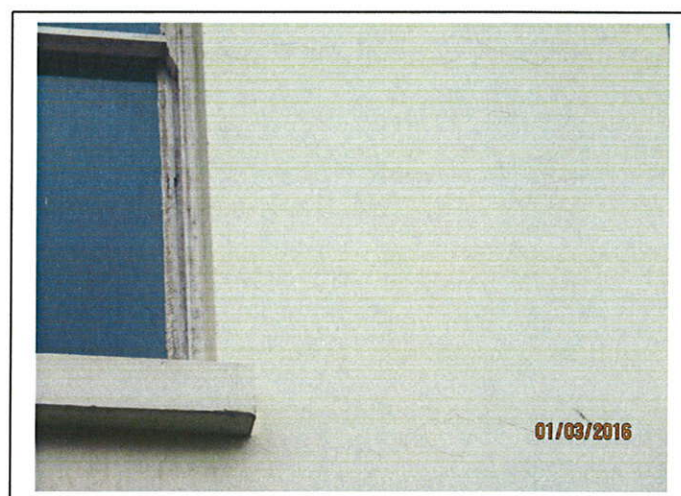
Typical cracking in render.
