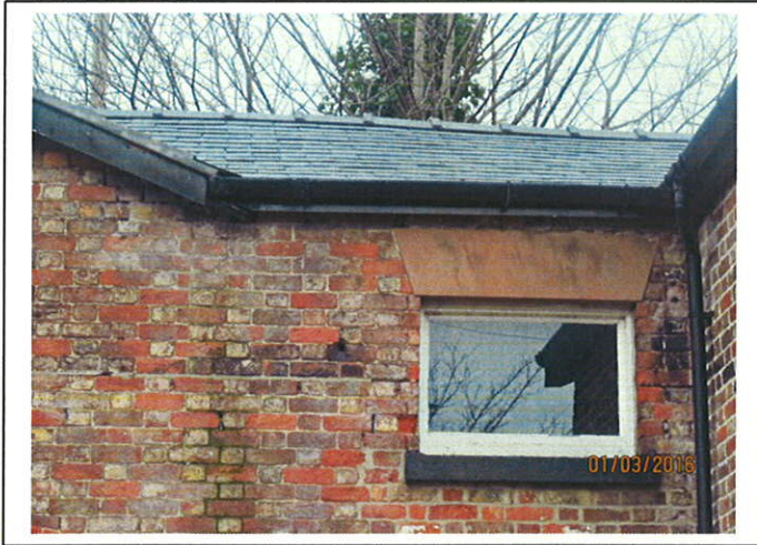
Roof deformation.
