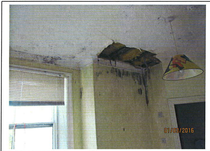
First Floor Room 14 - Damp penetration causing collapse to ceiling.
