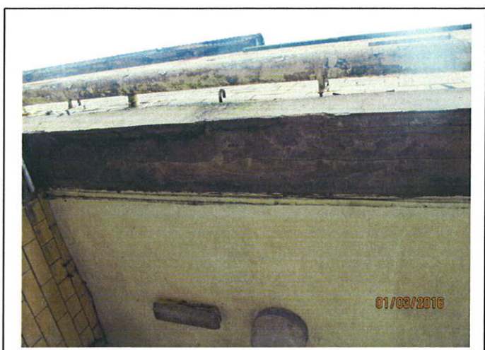
Spalled concrete lintel.
