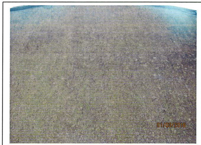
Right hand elevation Day joint in render.
