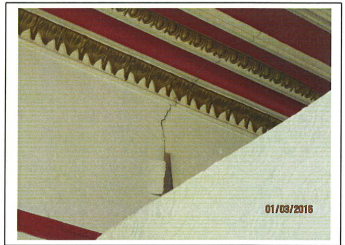
Ground Floor Room 8 - Staining on the chimney breast.
