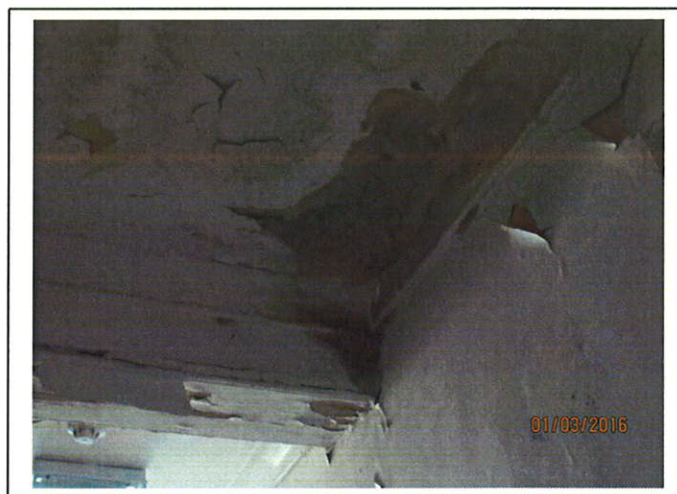
First Floor Corridor in front of Room 9 - Damp penetration through ceiling.
