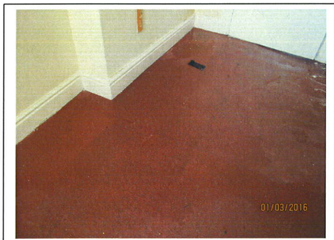
First Floor Room 15 - Ponding from leaking roof.
