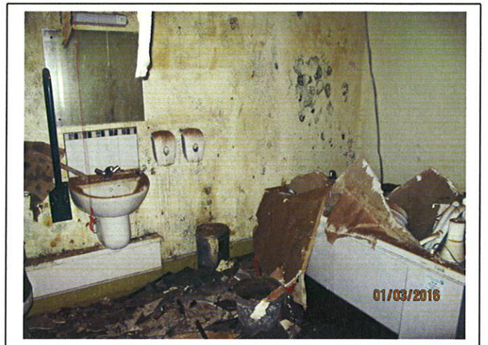
Ground Floor Room 22 - Water damage to bathroom
