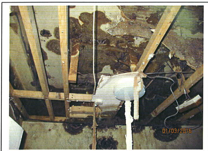
Ground Floor Room 22 - Water damage to bathroom.
