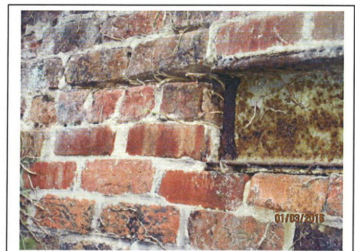
Corroded steel over window in rear elevation.
