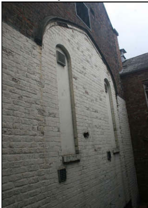
Original gable wall showing outline of west window and cast iron hood mould
