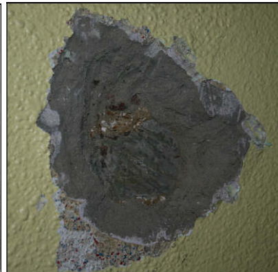
Modern plaster facing to original walls of church
