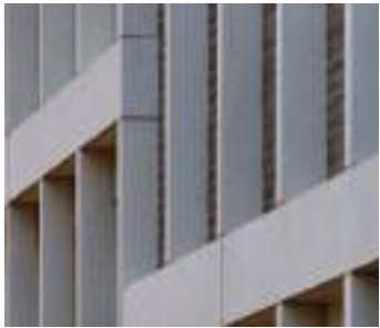
Light grey stone / concrete horizontal bands / entrance portal
