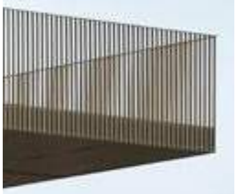
Flat plate steel balustrade to balconies and roof terraces
