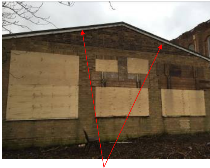
Gaps between fascia & brickwork to adjacent structure
