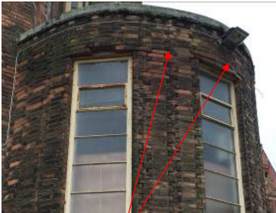
Crevice within brickwork
