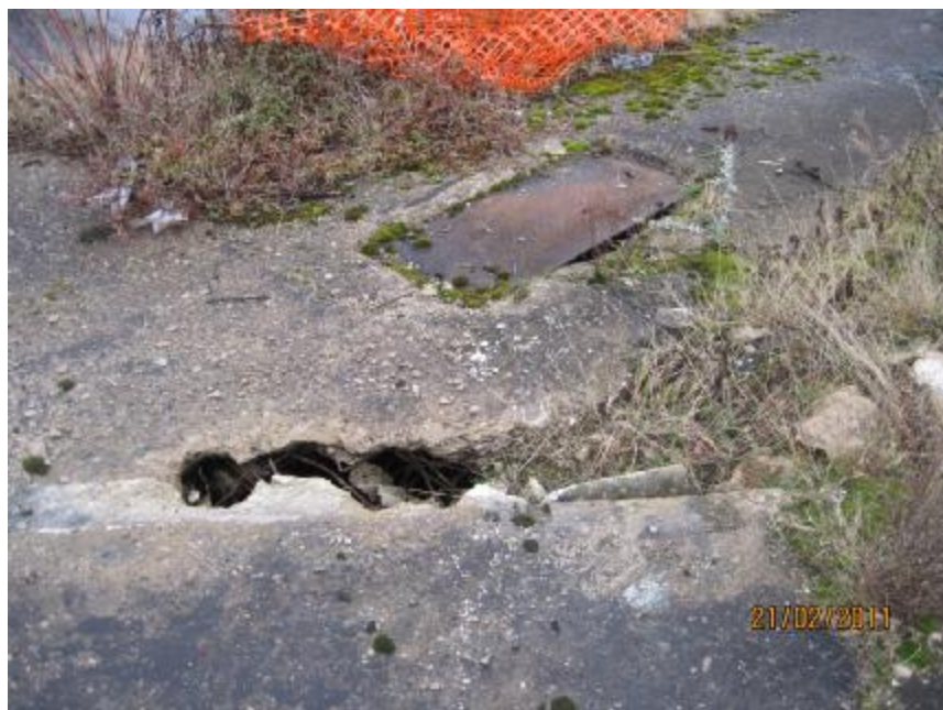
Plate 6: Void exposing metal pipes beneath reinforced concrete hardstanding
