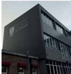
Recent overclad of front elevation of existing school building on site
