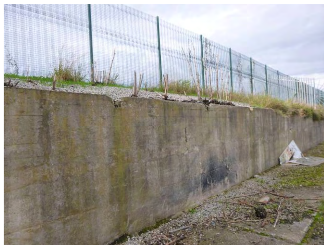
Retaining wall for hardstanding sports surface at southern end of site. Note treated dead stems of Japanese knotweed on top of wall.
