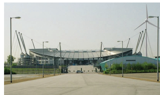
Figure 4-4: The scrapped 360ft wind turbine at the Manchester Sportcity development
