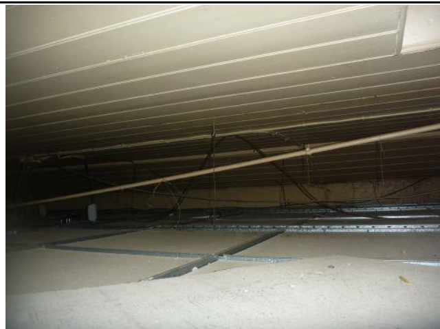
Photo 9.25: Building 1, section 1c showing vaulted ceiling above suspended ceiling.
