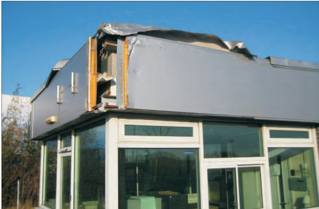
PHOTOGRAPH 3: Damage to Roof of Building B3
