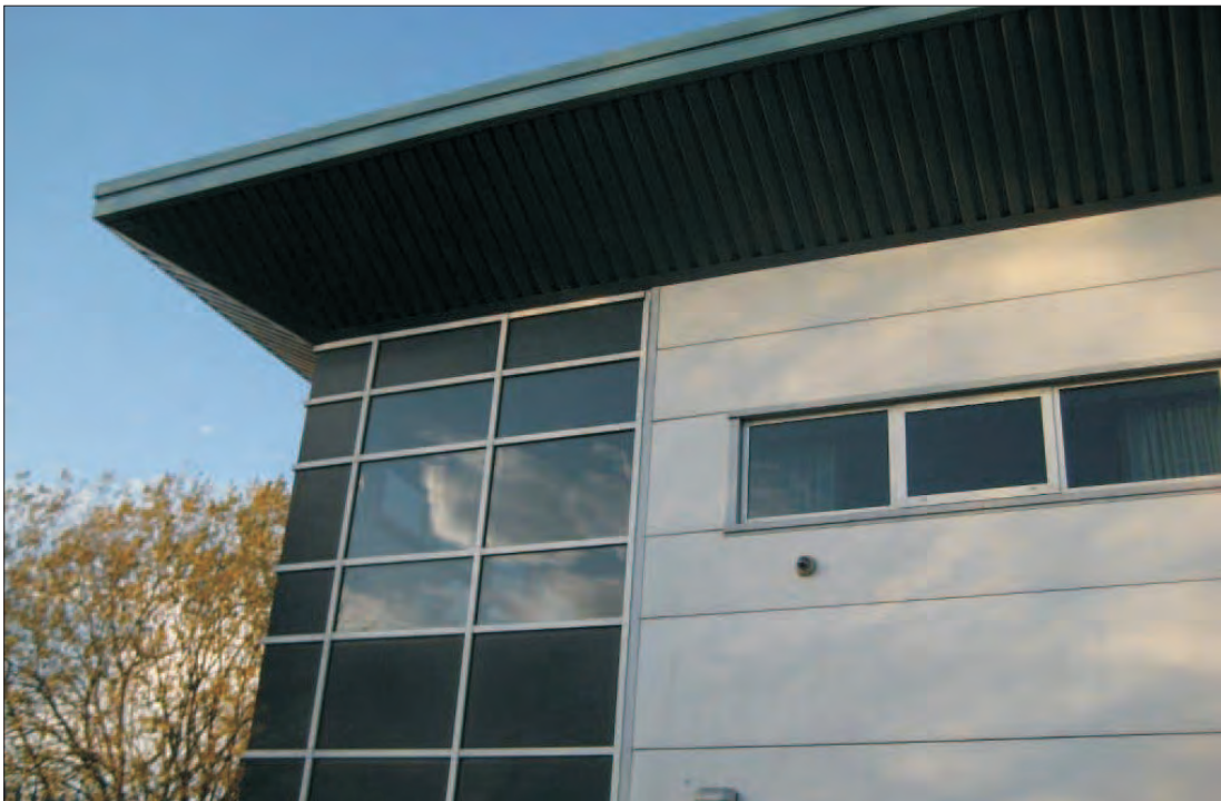
PHOTOGRAPH 6: View of Building B4 Showing Crevices in Frame / Cladding
