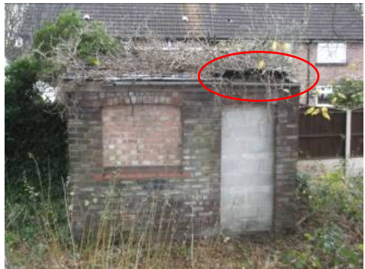
Building A with collapsed slates
