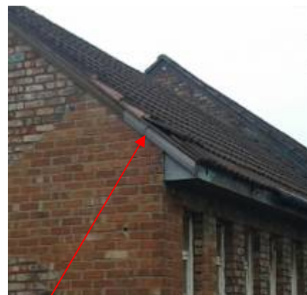
Lifted roof tiles on Building B
