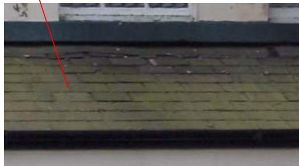
Gaps where the tiles have slipped
