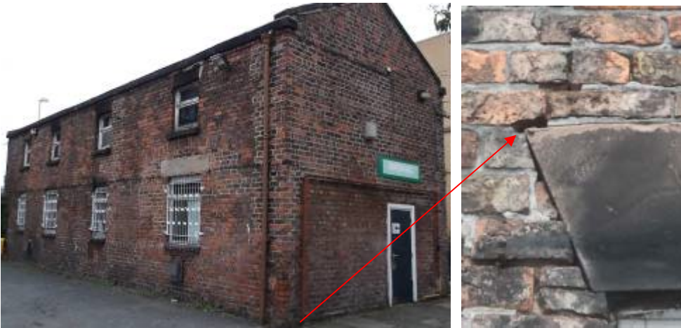
Building J – Viewed from south-west, gaps in brickwork
