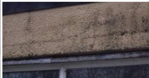
Building K - Viewed from south-west, gaps between concrete roof and flashing
