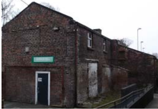
Building J – Viewed from south-west, gaps in brickwork
