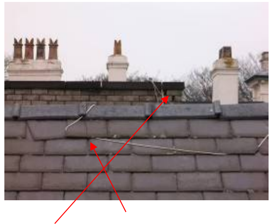
Gaps in brickwork and roofing tiles
