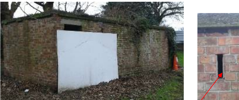
Building M - Gaps in brickwork on north-east and south-west elevations
